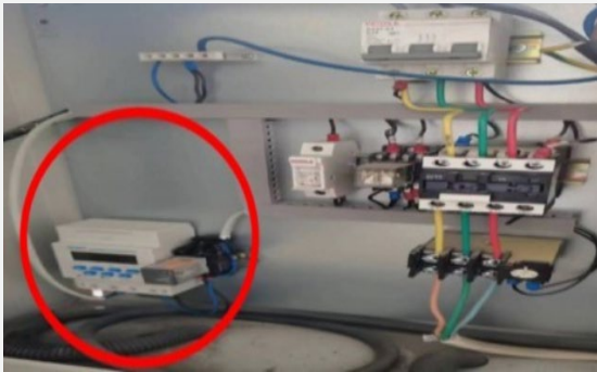
Electrical Upgrades on Workshop Doors
